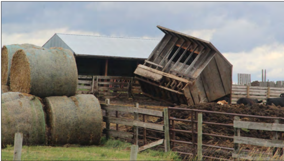
Farm buildings were badly damaged by the high winds.
