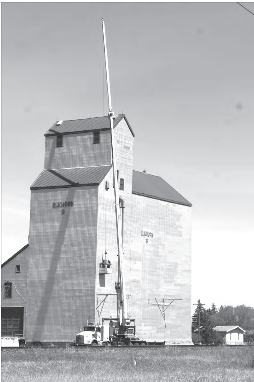
Elkhorn elevator repair day.
