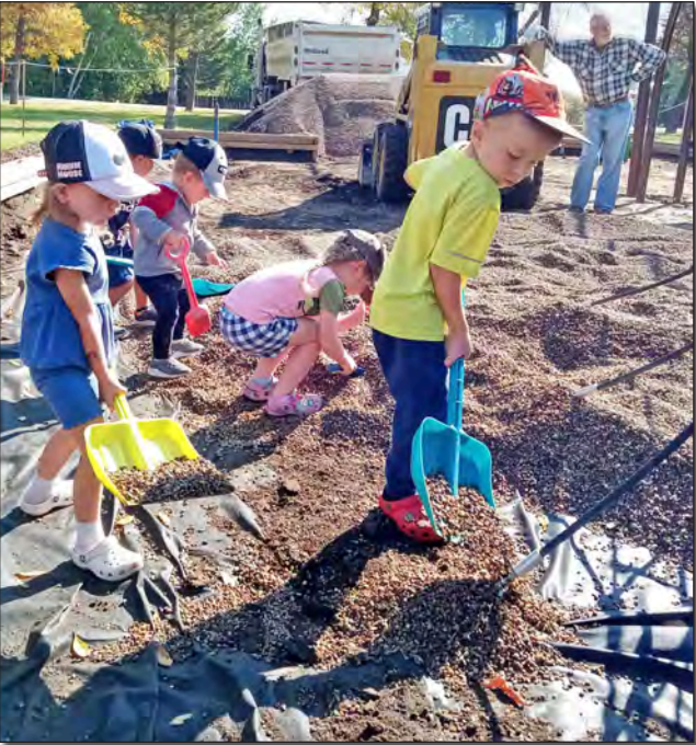
Young enthusiasts help to distribute the gravel into the play structure base.
