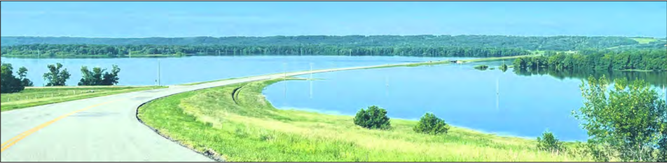
The PR 259 heading towards Virden sees water very close to the highway.
