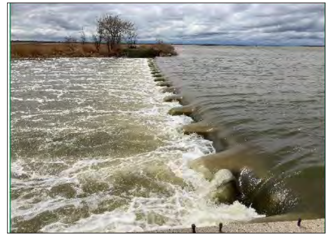
Oak Lake Dam weir structure.
