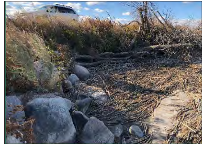
East dike to be rehabilitated.
